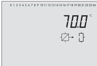
Flow sensor VF2, DHW circuit
