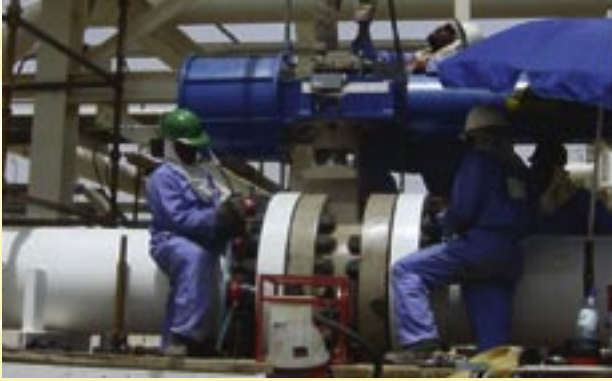
Assembly of the LEUSCH butterfly valves in the Sultanate of Oman. · All the products manufactured by LEUSCH have a high technical standard and have been extensively tested at all manufacturing levels. Like SAMSON, LEUSCH is certified according to ISO 9001:2000.
