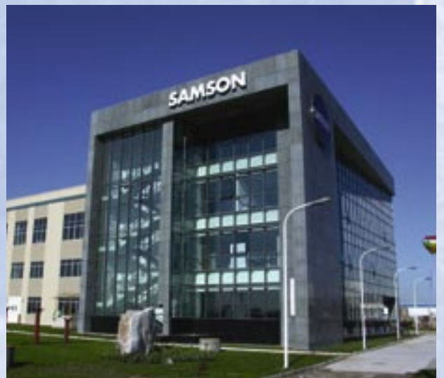
The new four-story head office of SAMSON CONTROLS (China) Co. Ltd. in the Beijing Economic Technological Development Area (BDA).
